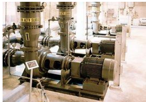
Figure 9. Grundfos horizontal dry-pit sewage pumps.
