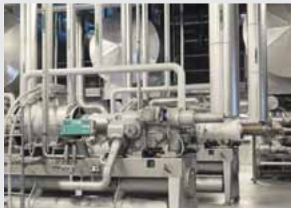
Fig. 9: Piston compressor
