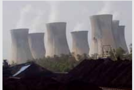
Cooling towers at a coal fired power plant
