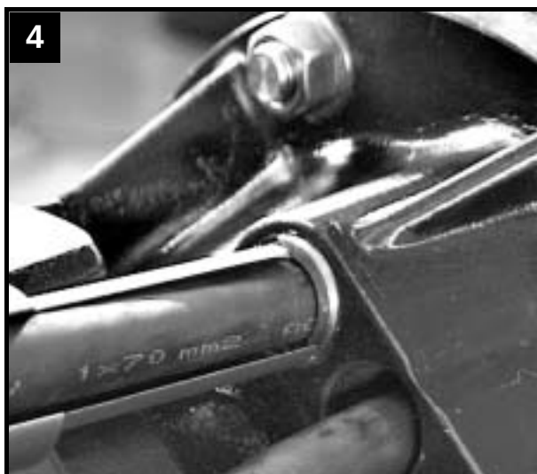
Tighten cable glands with special tool
