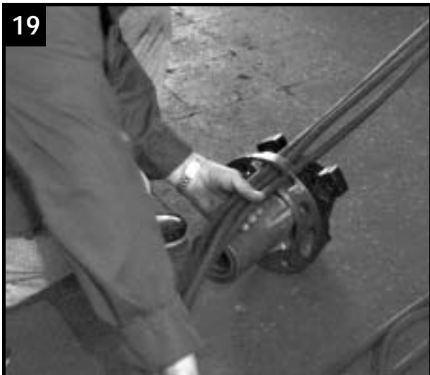
19 Pull cables through upper bearing housing
