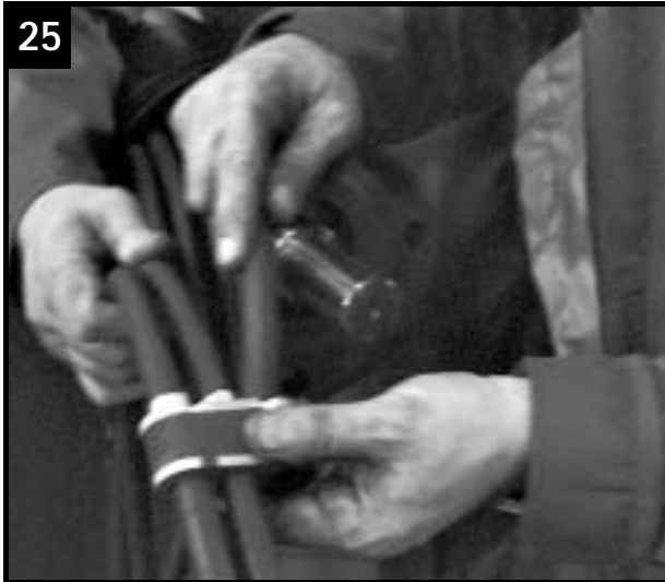
25 Pull cables through cable gland ring and grommet
