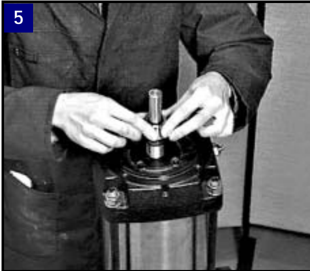
5 Fit shaft seal and press it into bottom position without use of any tools.
